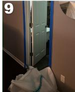
This photo shows a door containment that has fallen completely before the PRV.
