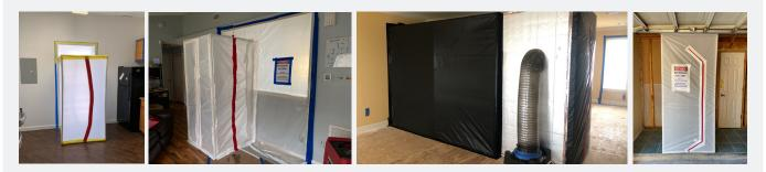
These photos show a decontamination chamber, which is designed so that mold technicians can decontaminate themselves prior to leaving the job site. That being said, if your technicians are able to exit the work area directly to the outside of the building, then a decontamination chamber is not necessary.
