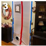
The containment barrier in this photo is an example of how the contractor used a filter for make-up air. Additionally, it demonstrates how the contractor used an air filtration device to install negative air — by setting up the output to be exhausted from the work area.
