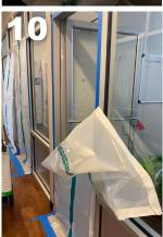
This photo shows a door containment that was partially separated from the door trim prior to the PRV.
