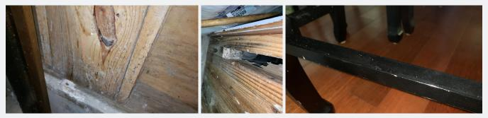
All of these photos are examples of what not to do with regard to the cleanliness of the job site. Oftentimes, instances like these occur when technicians — especially those that are new to the industry — forget to clean inside wall cavities, on wood framing, and/or on horizontal surfaces of furniture prior to LAQ's PRV inspection.
